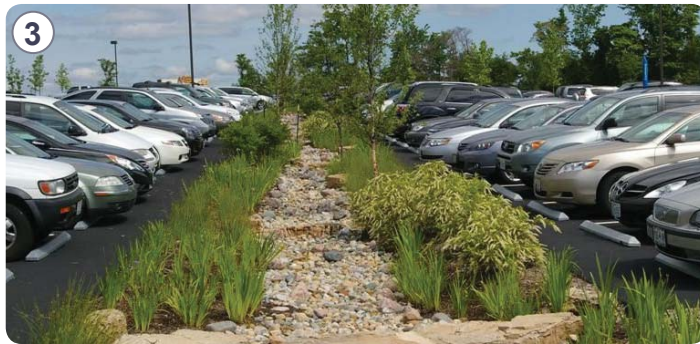
WSUD swales to collect and filter stormwater runoff
